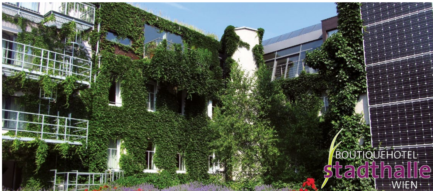
© ASSA ABLOY Entrance Systems AAES_Referenz_Boutiquehotel Stadthalle Wien_2018
