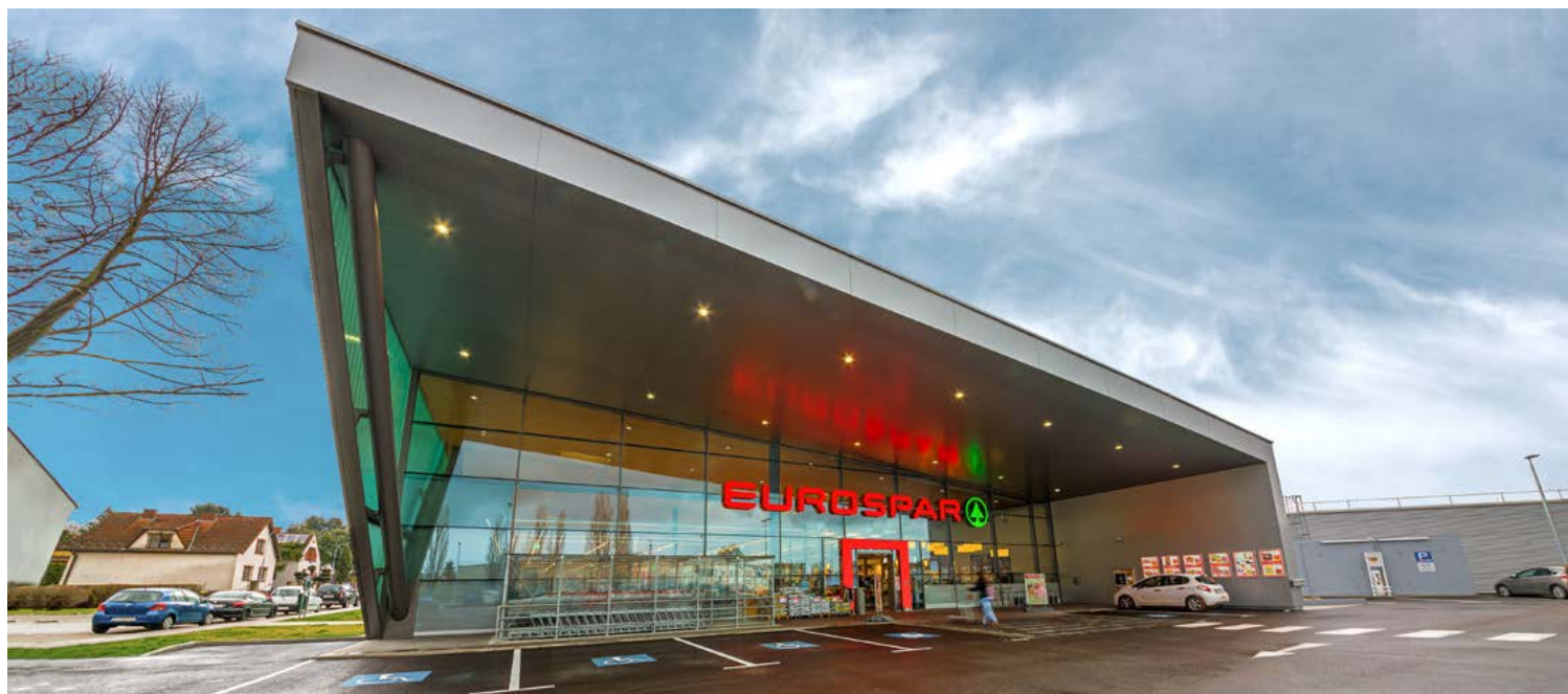
© ASSA ABLOY Entrance Systems AAES_Referenz_Spar_2019
